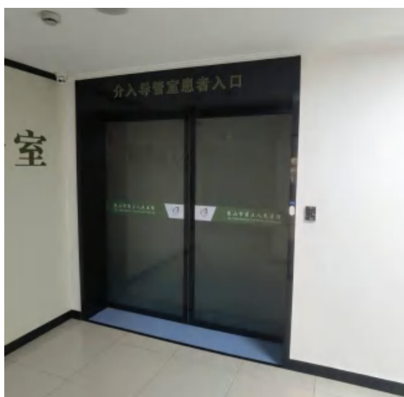
DSA 机房西侧缓冲间
